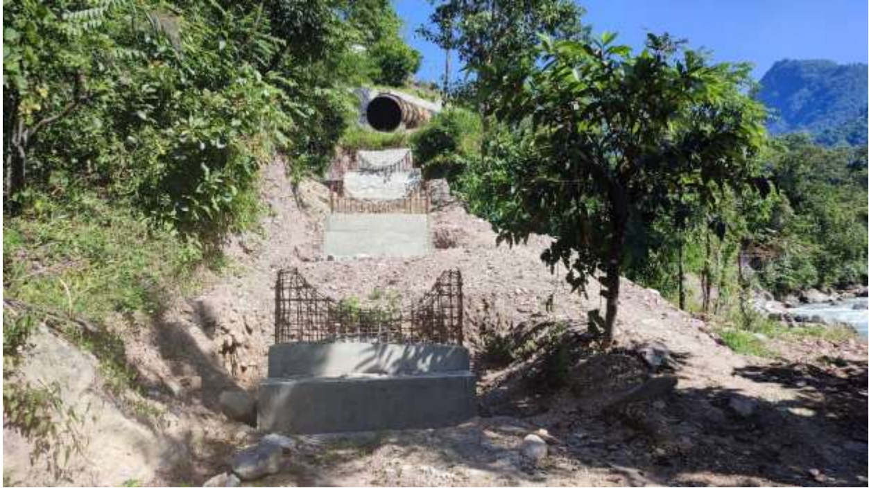
Saddle support rebar works between IP21-IP22
