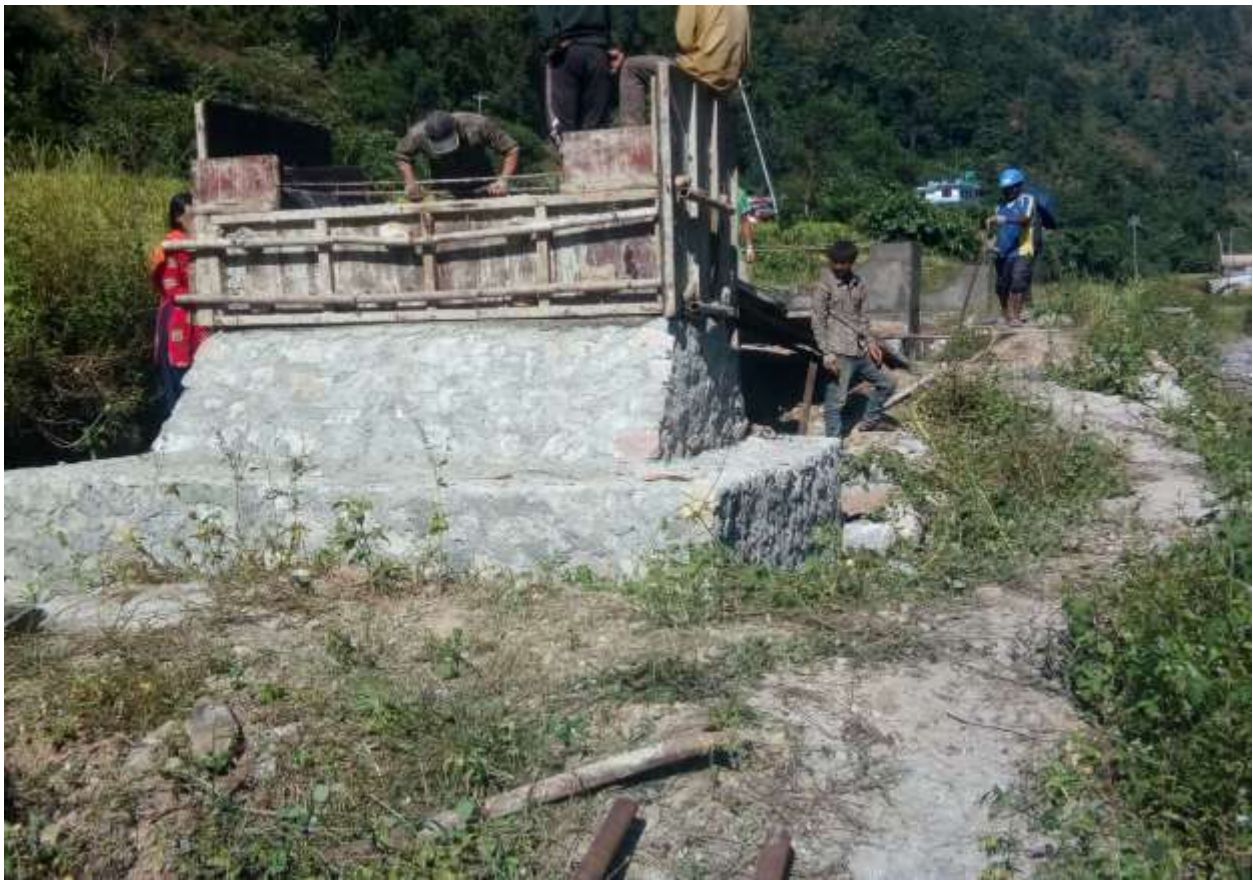
Saddle support formworks
