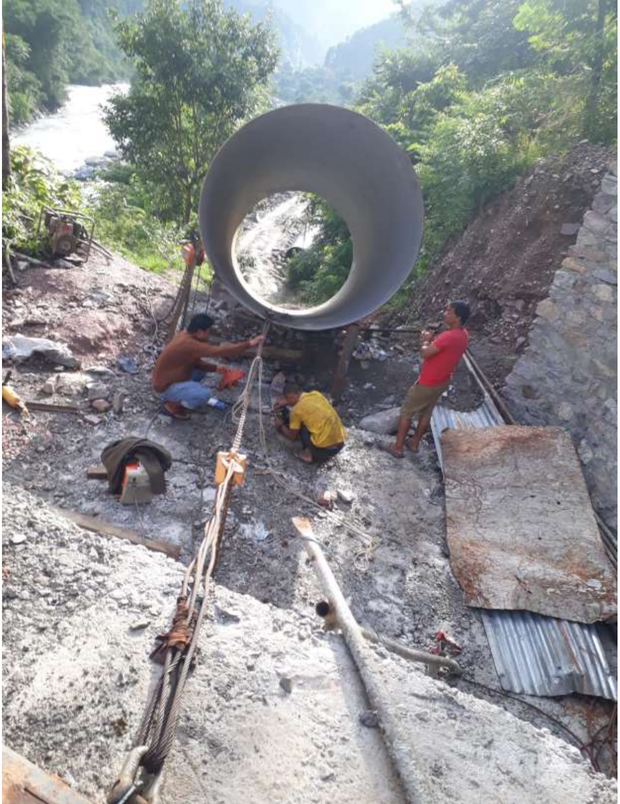
IP21 Bend erection
