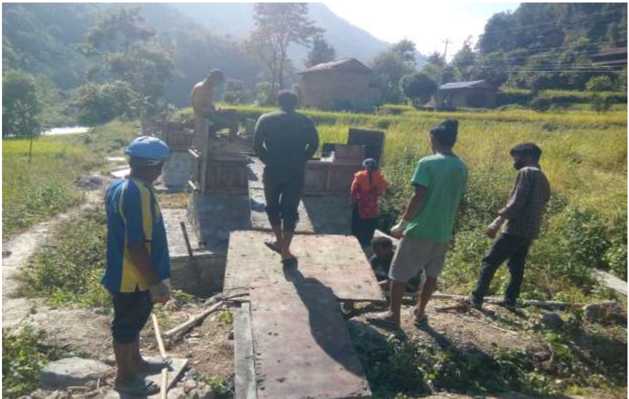
Saddle support 2 nd lift concreting between IP28-IP29
