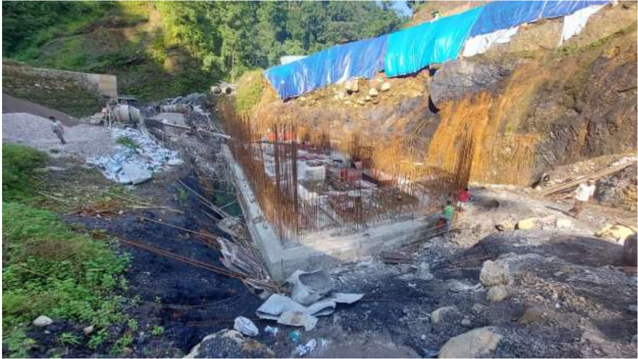
Rebar works for powerhouse shear wall
