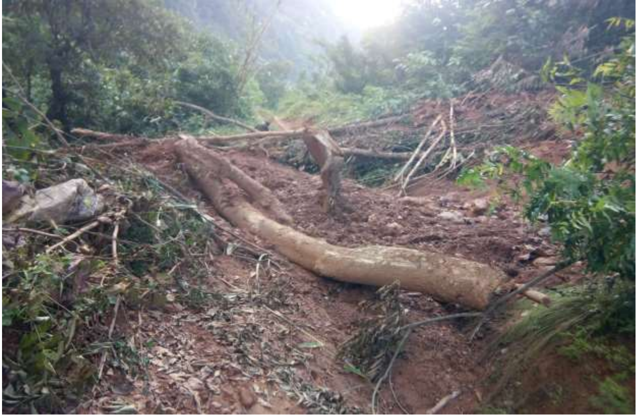
Landslide at Surge Tank
