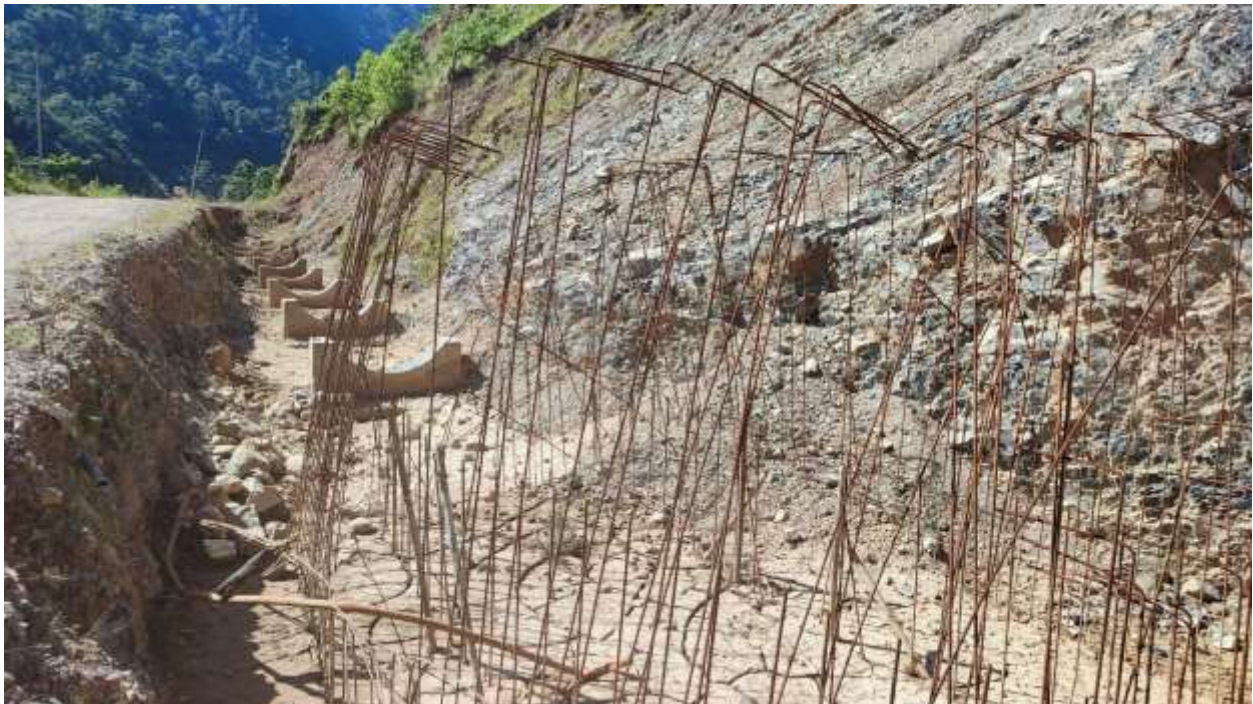
Site clearance between IP48-IP49
