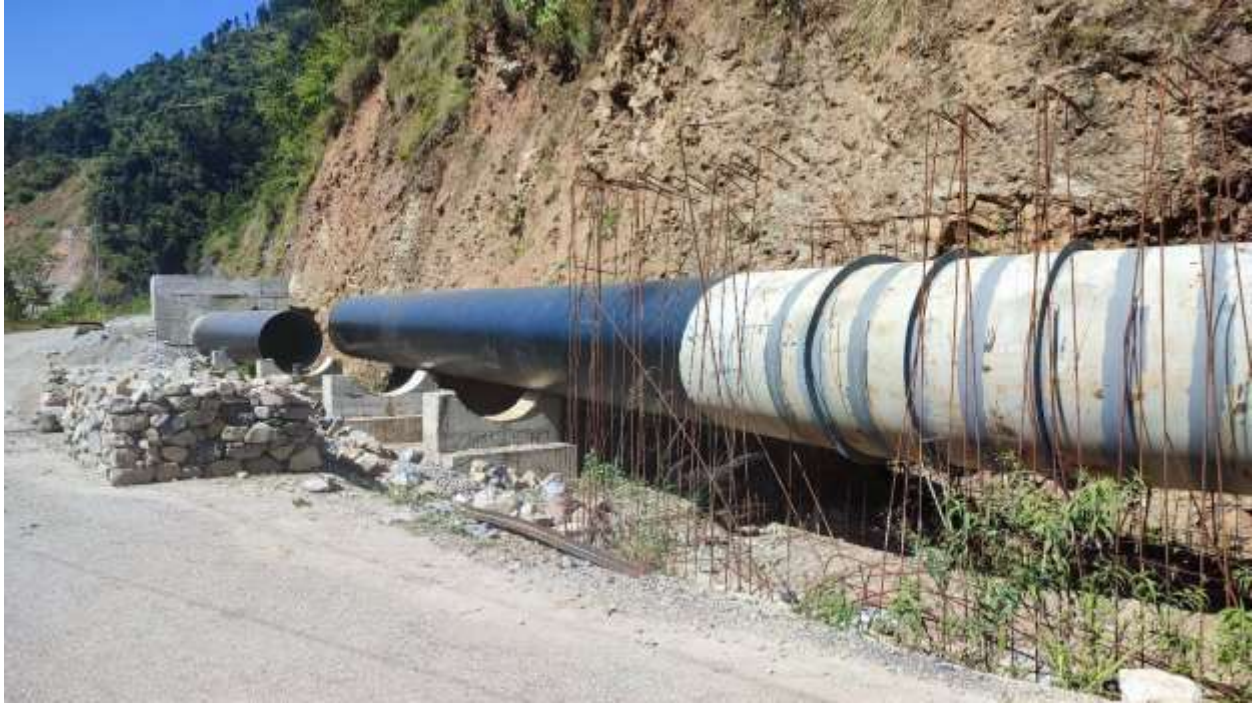
Pipe erection between IP43-IP44
