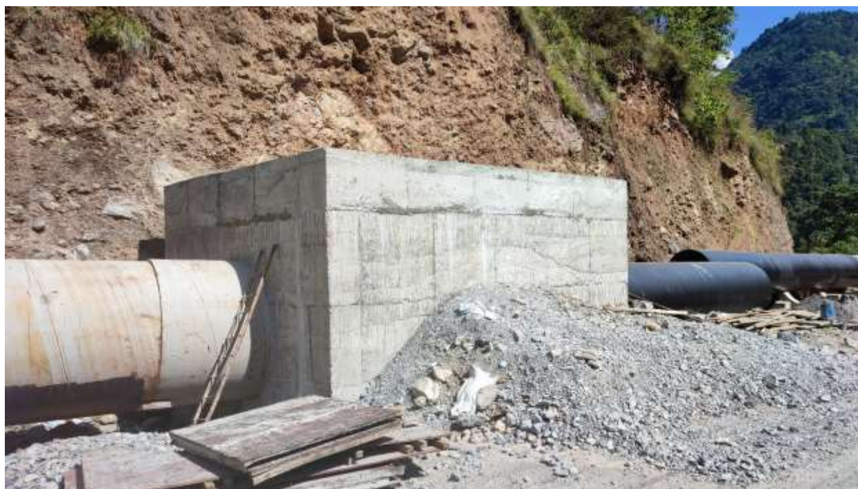
AB44 after completion
