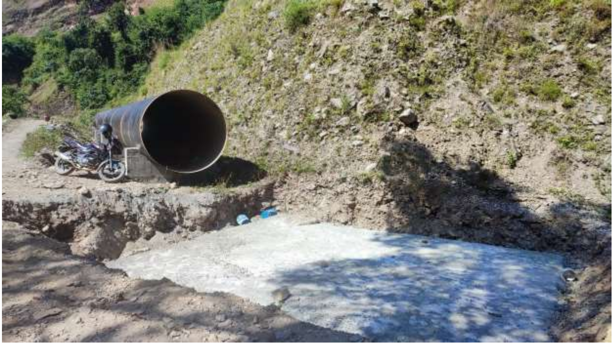
Pipe erection between IP9-IP10
