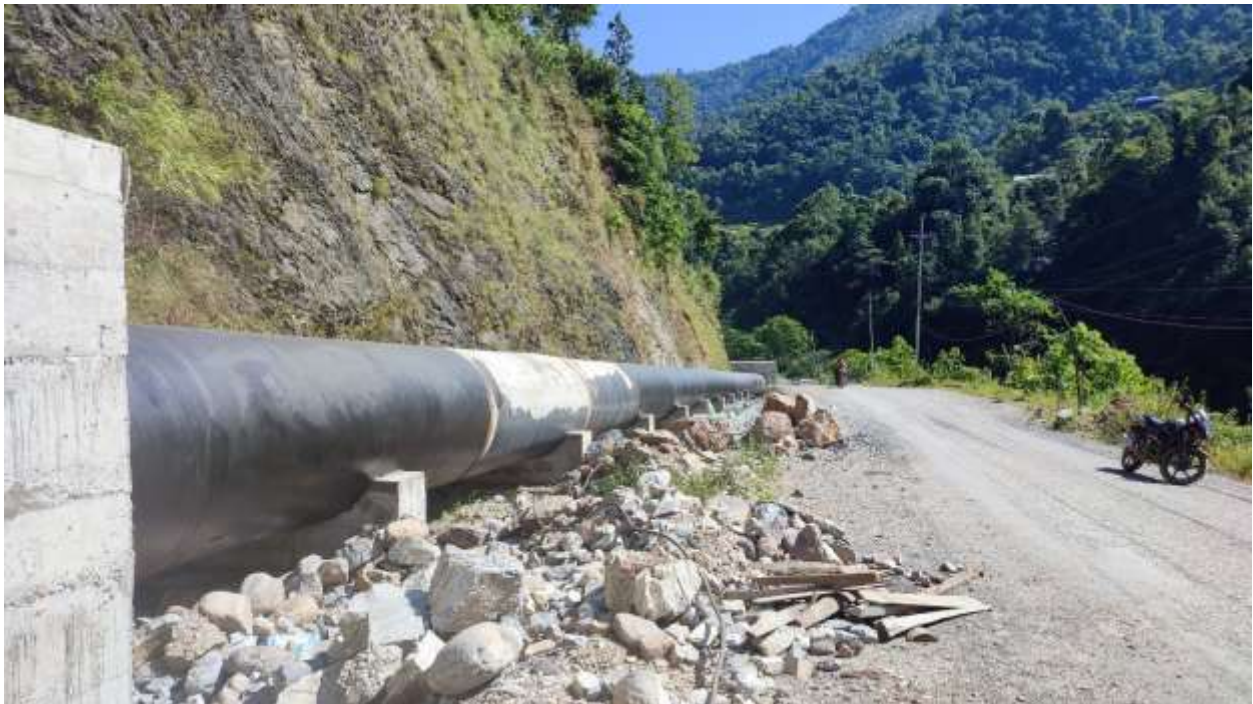
Pipe erection between IP44-IP45
