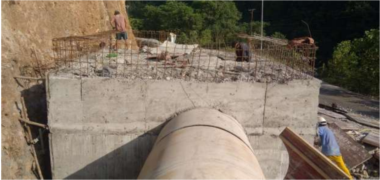
AB44 Rebar works
