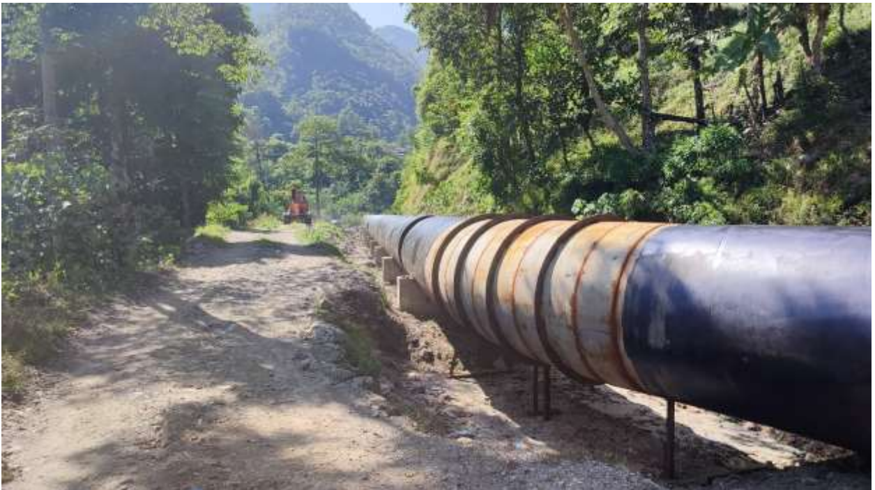
Pipe erection between IP-IP9
