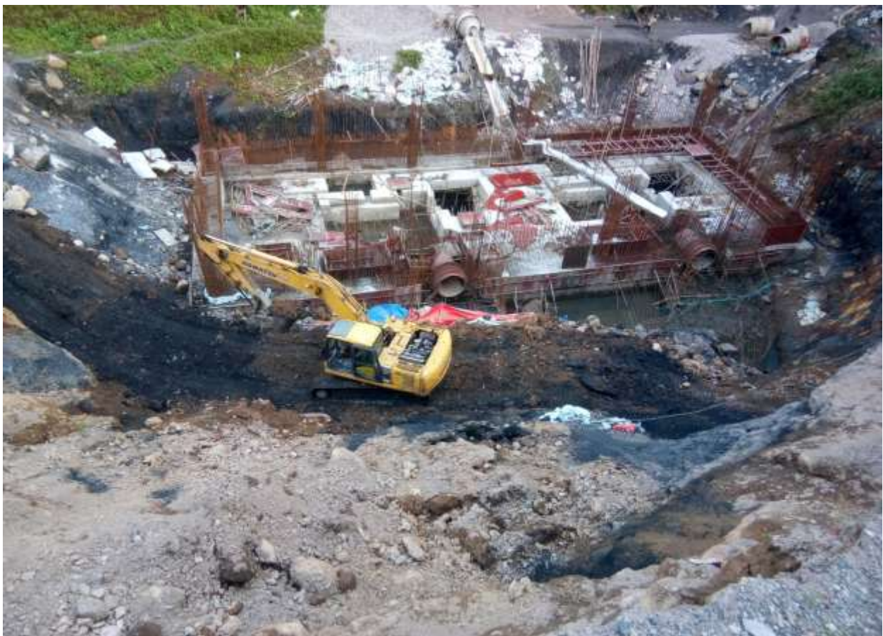
Landslide clearance at powerhouse
