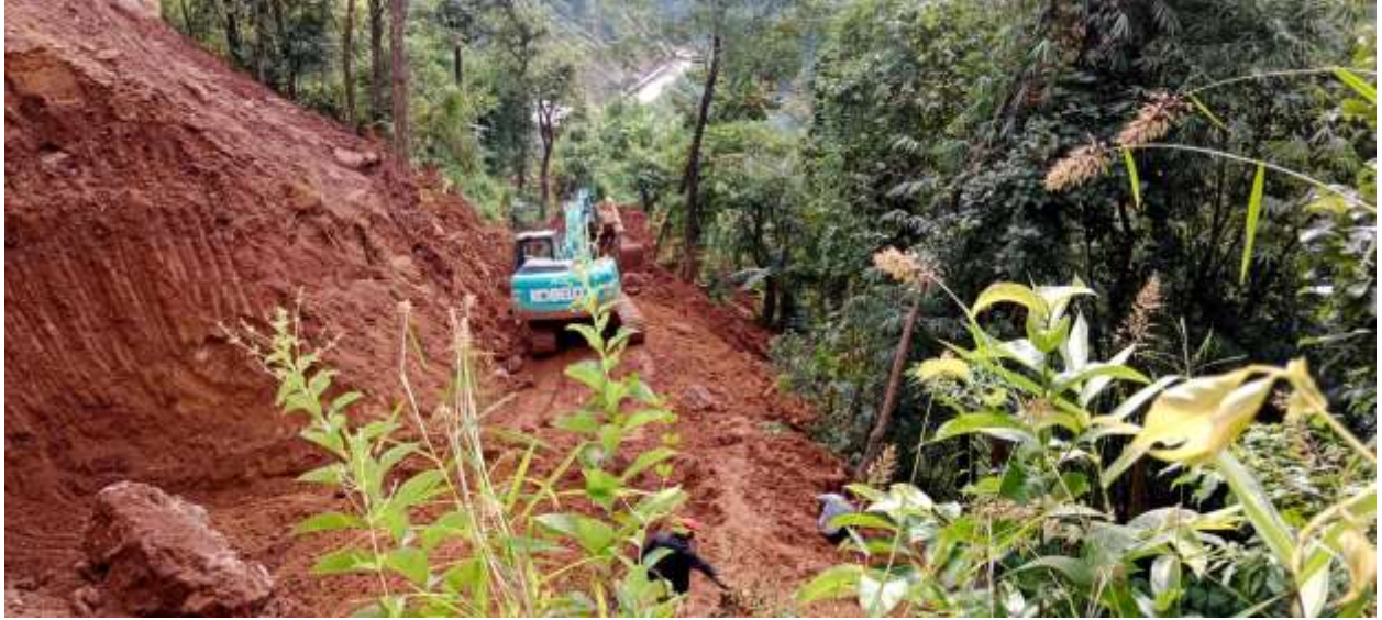
Surge Tank excavation works I
