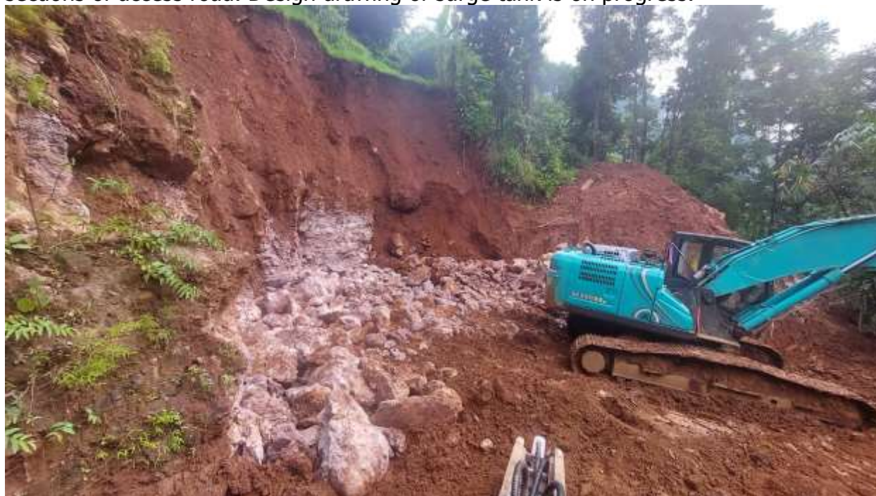
Surge Tank excavation works
