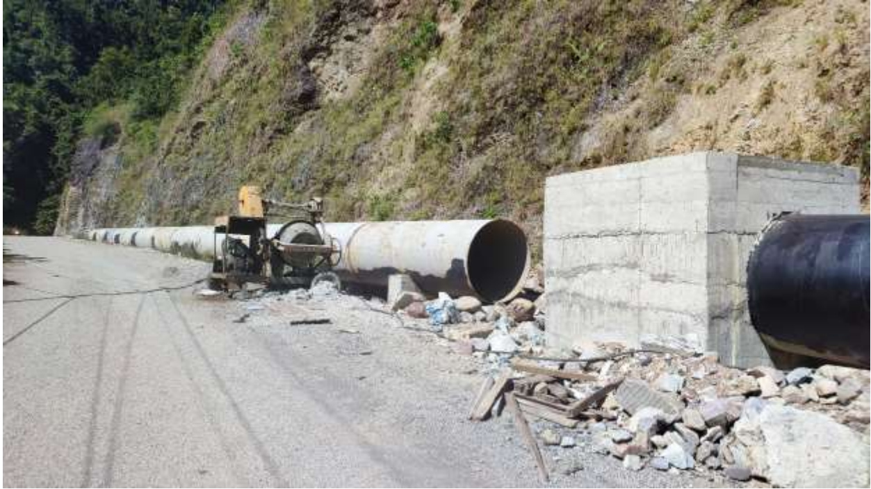
Pipe erection between IP45-IP46
