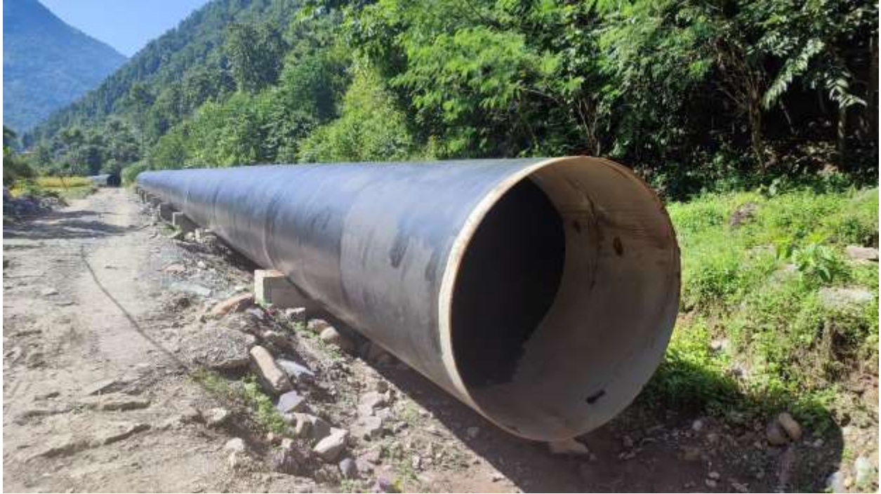
Pipe erection between IP22-IP24
