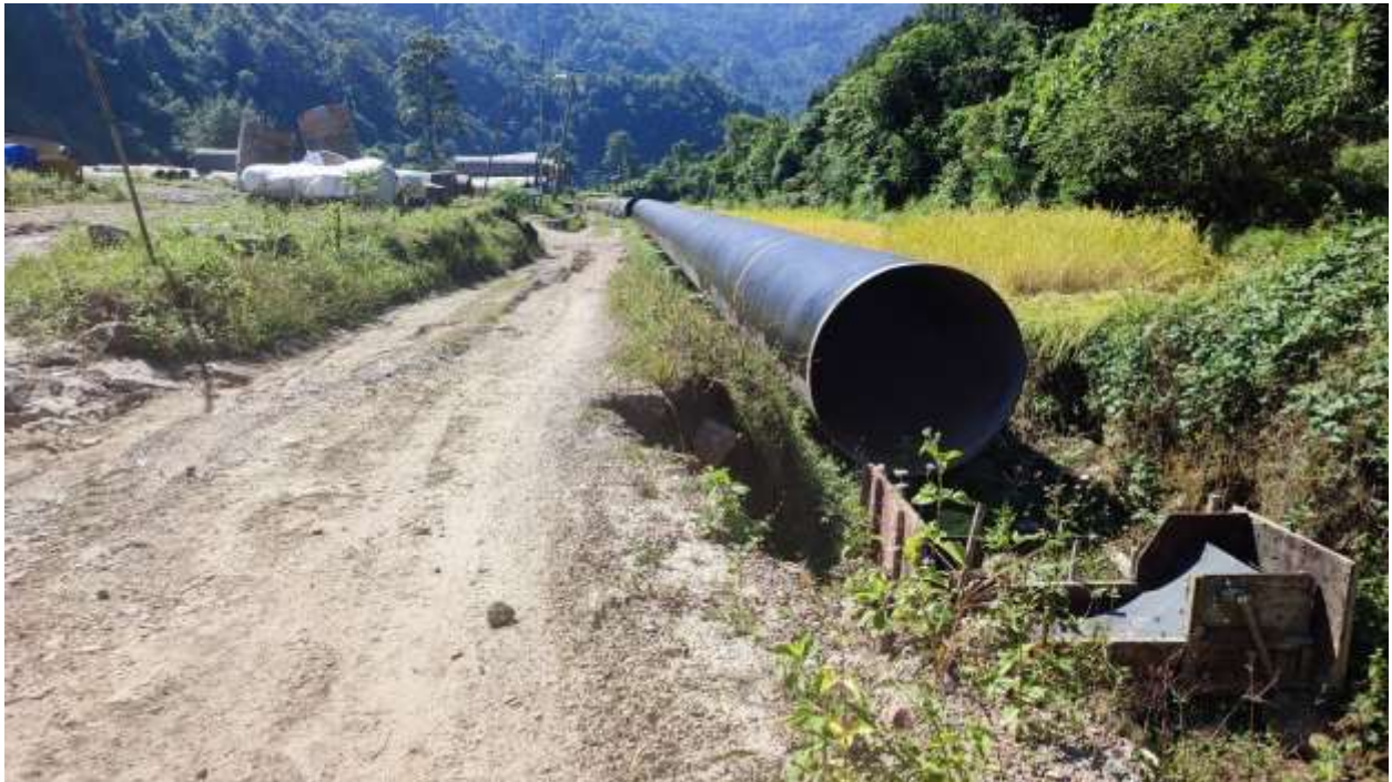
Pipe erection between IP25-IP27
