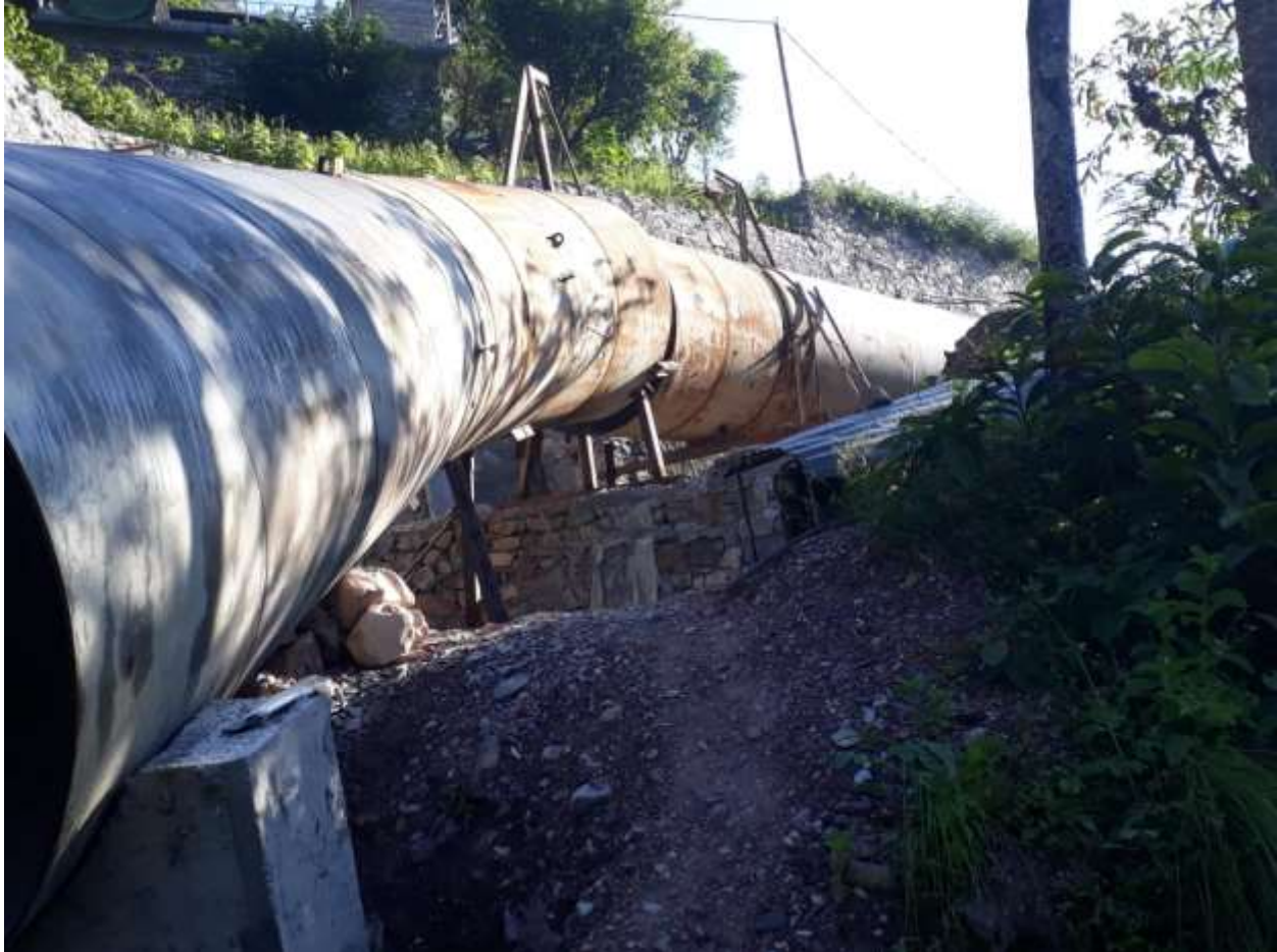
IP21 Bend erection
