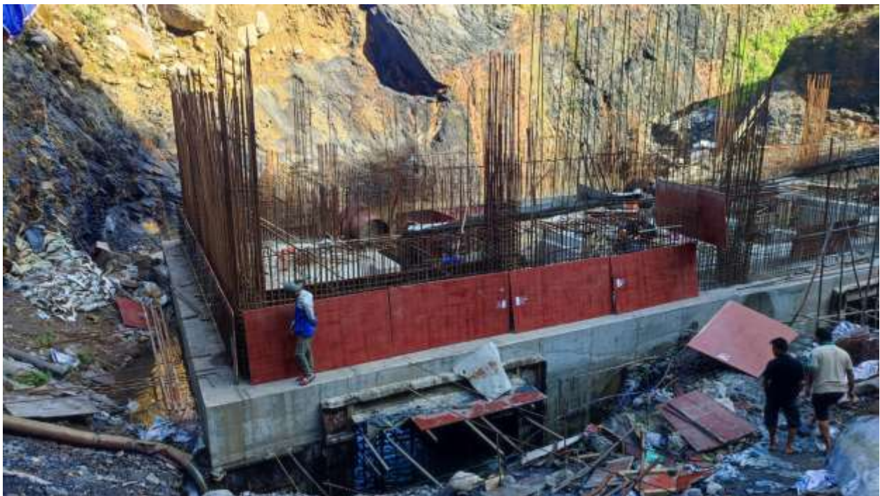
Formworks for powerhouse shear wall
