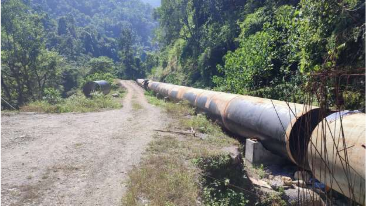
Pipe erection between IP6-IP8
