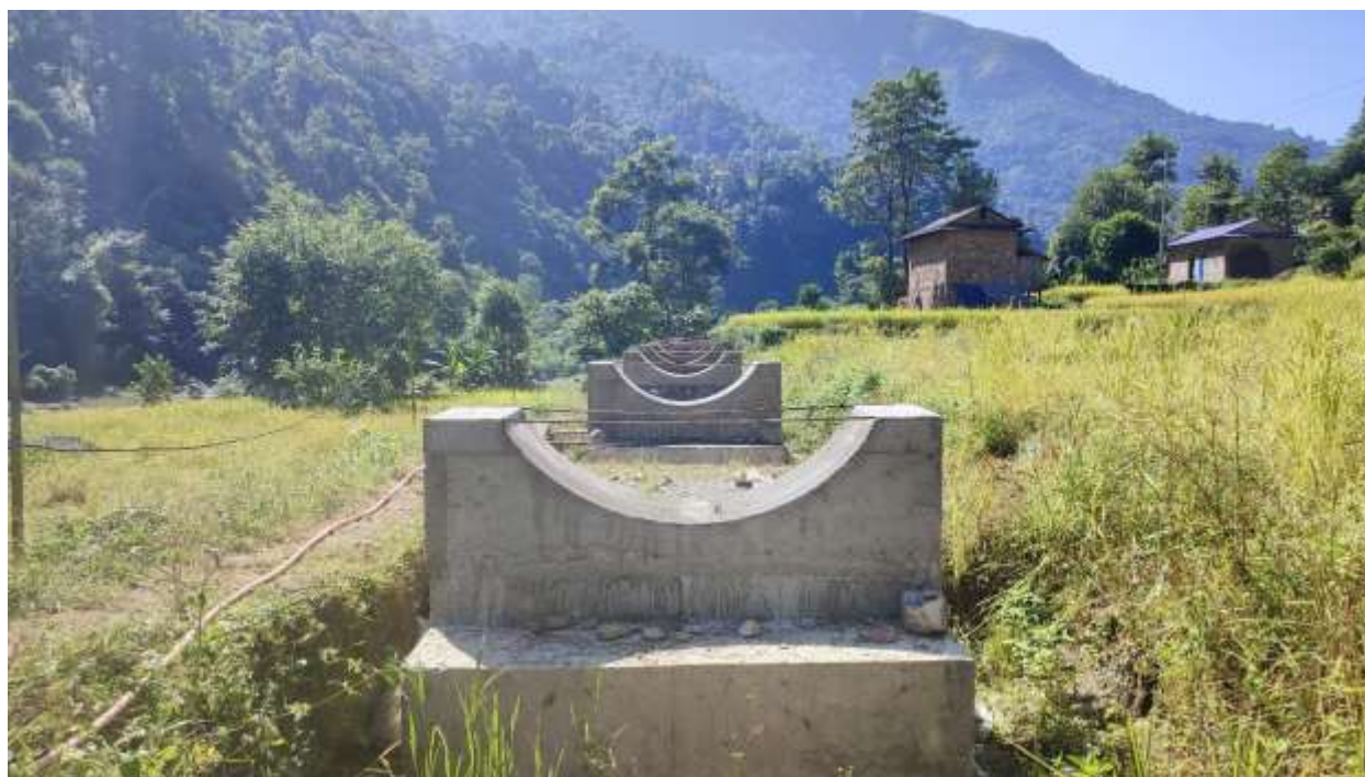
Saddle support works between IP28-IP29
