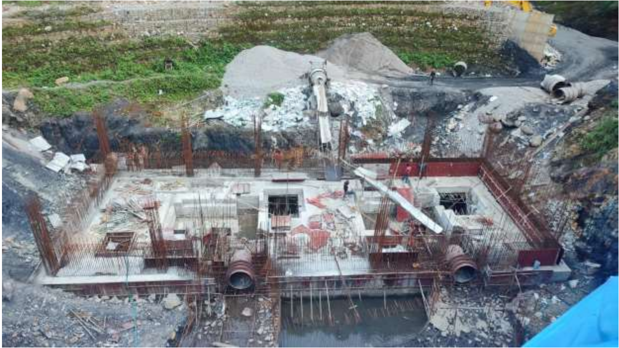
Powerhouse Top View
