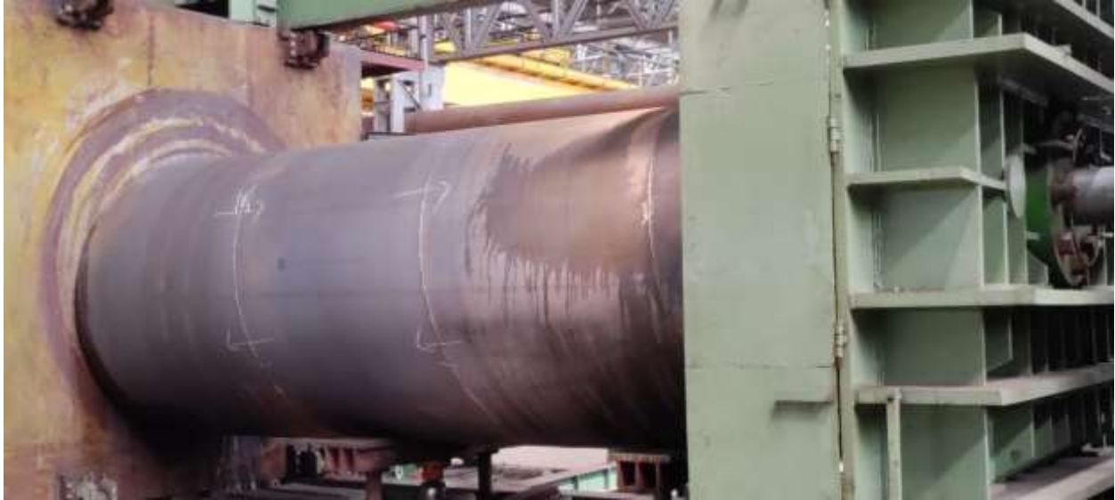
2 nd lot pipe rolling works at Factory
