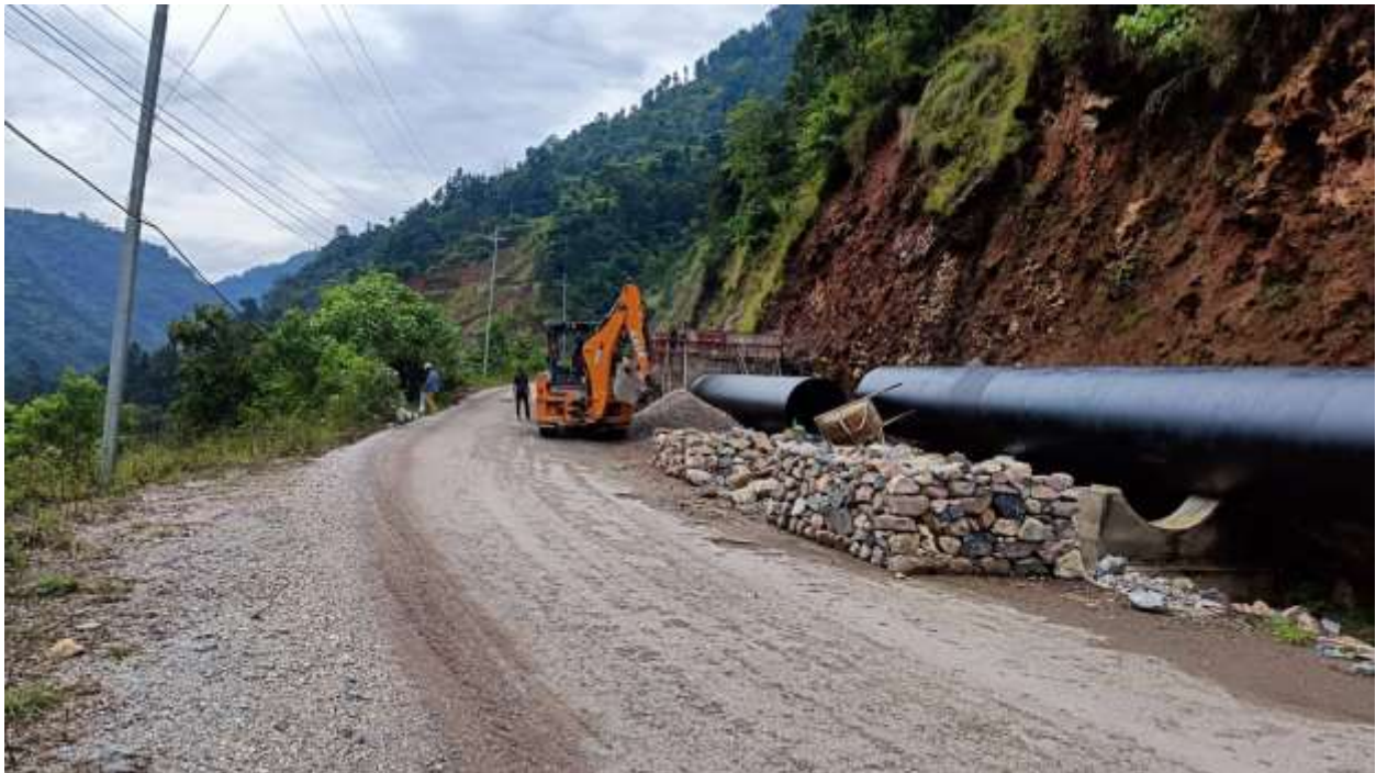
Anchor Block 44 concreting works
