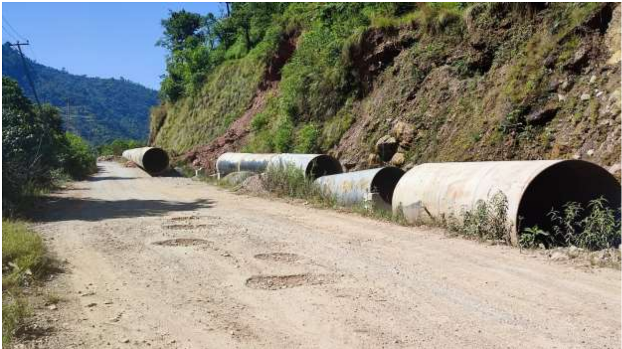
Pipe erection between IP42-IP43
