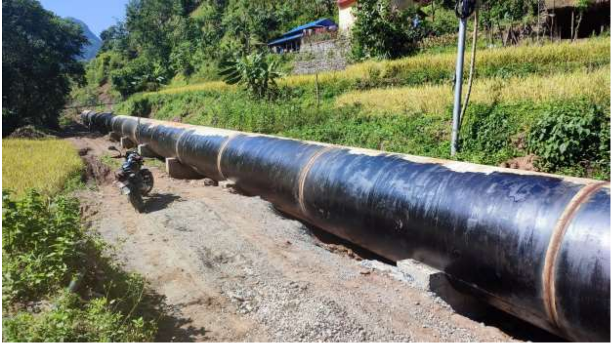
Pipe erection between IP35-IP36
