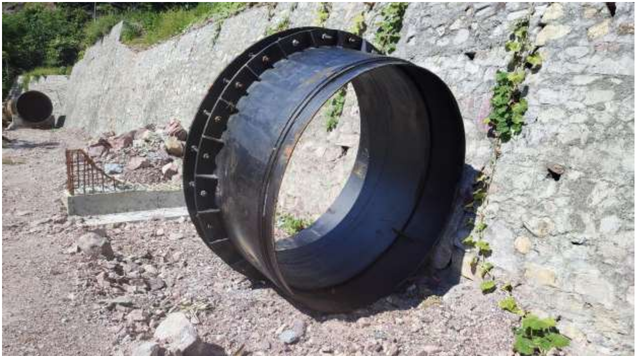
2100mm dia. Expansion joint unloaded at site
