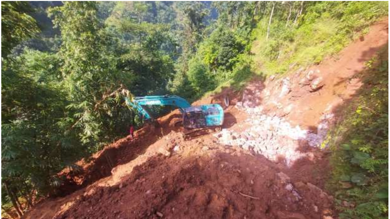
Surge Tank excavation works II
